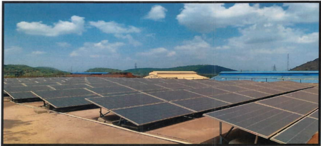
Solar Panel Capacity 72 K.W at Roof top of CDSS Building.
