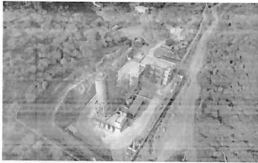
Hydro Fill Plant
