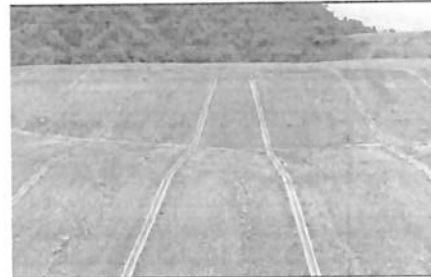
Tailing Embankment Drain
