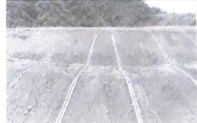
Tailing Embankment Drain
