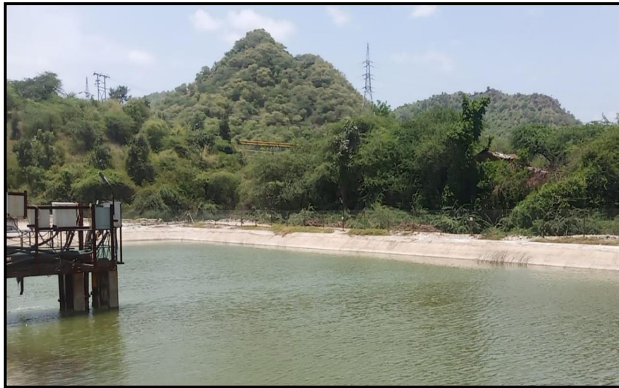
Recycling arrangement (storage cum pumping arrangement)
