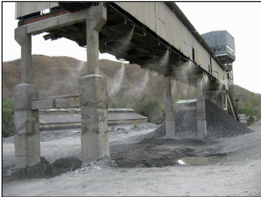
Mochia Coarse Ore Stockpile
