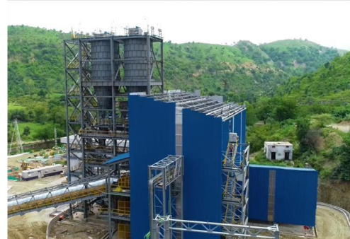
Paste Fill Plant
