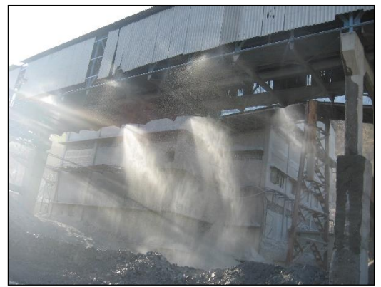
Balaria Coarse Ore Stockpile
