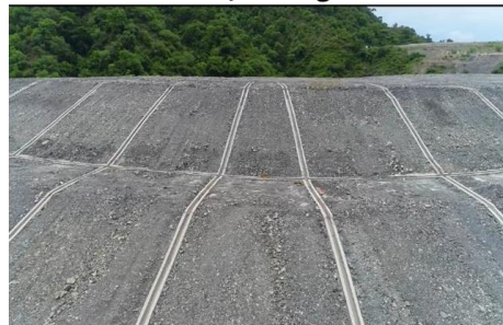
Tailing Embankment Drain
