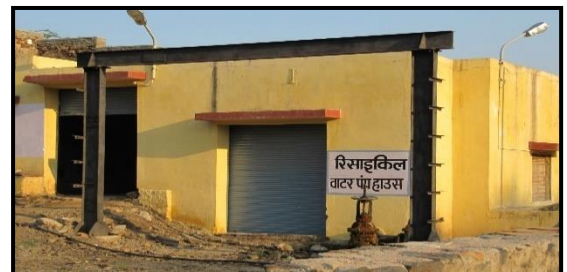
Recycling Water Pump House
