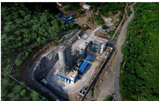
Hydro Fill Plant
