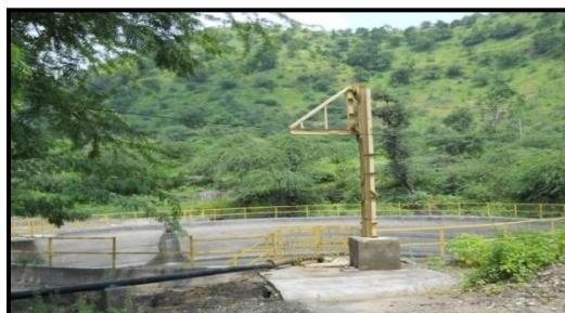
2,000 m 3 Capacity Water Reservoir
