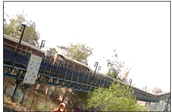
Covered Conveyor Belt
