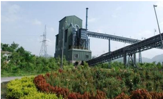
Covered conveyor belt
