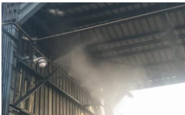
Mist sprinkling system in coal yard
