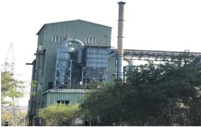
Coal Crusher Building
