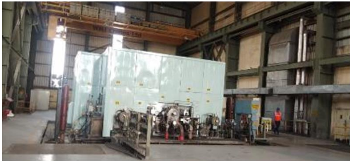
Acoustic Enclosure for Turbine
