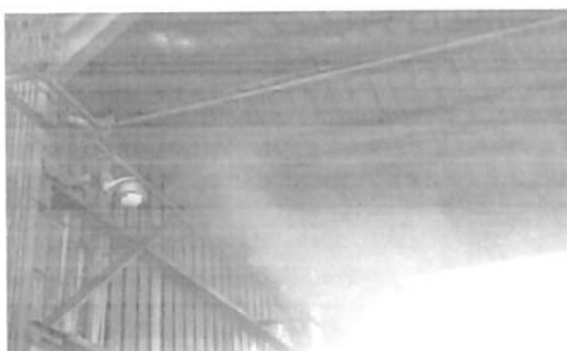
Mist sprinkling system in coal yard
