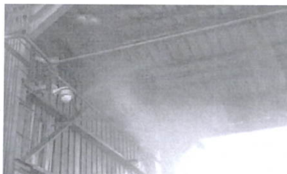
Mist sprinkling system in coal yard
