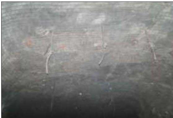
Development supported with Rock Bolt, Wire Mesh & Cable Bolt
