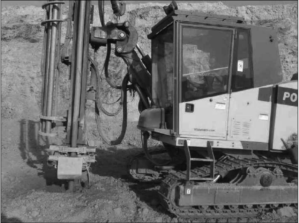
Fig : Wet Drilling
