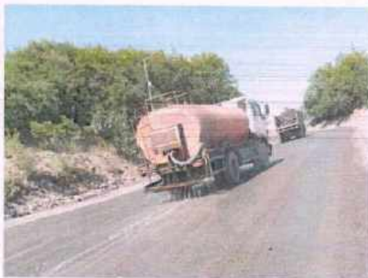
Water sprinkling on haul road
