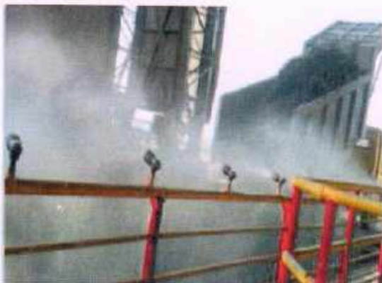
Auto dust suppression system at crusher
