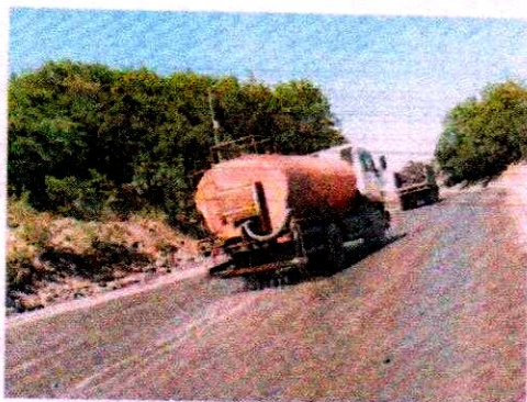
Water sprinkling on haul road
