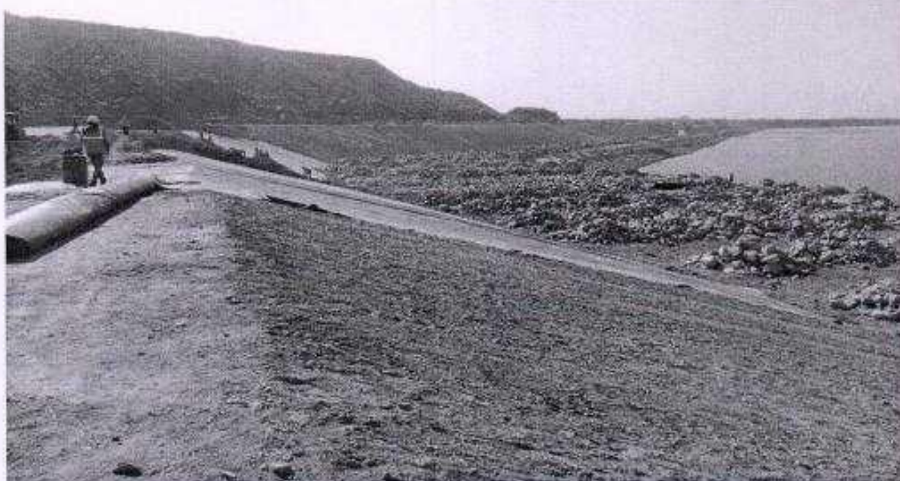
HDPE laying in tailing dam
