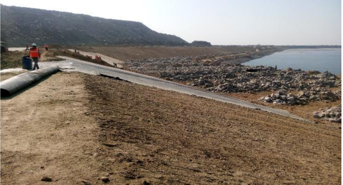
HDPE laying in tailing dam
