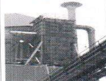
Bag filter, Cyclone at Coal Crusher
