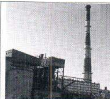
8 Field ESP with 165 mt Stack height
