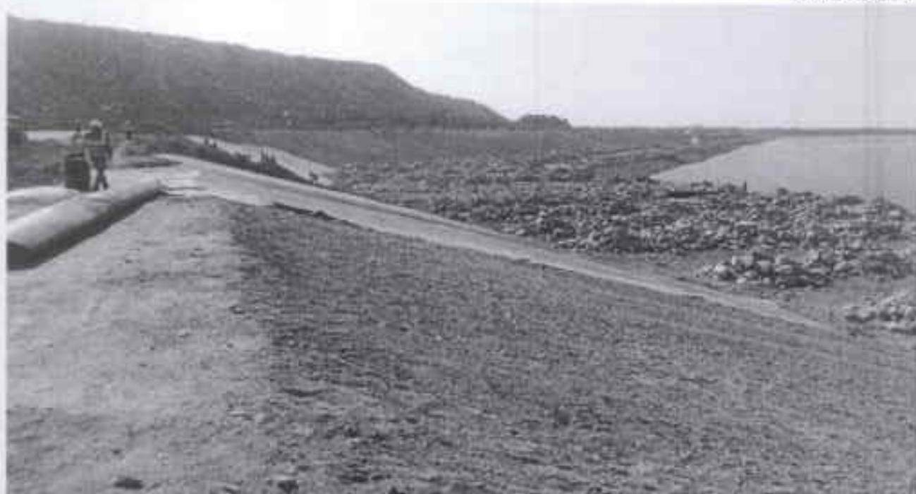
HDPE laying in tailing dam
