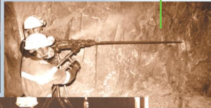
Drilling by hand- held hammer
