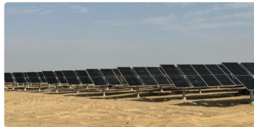
Modules installed at site
