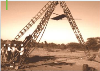
Conventional drill rig
