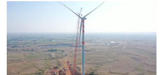
1st wind turbine installed
