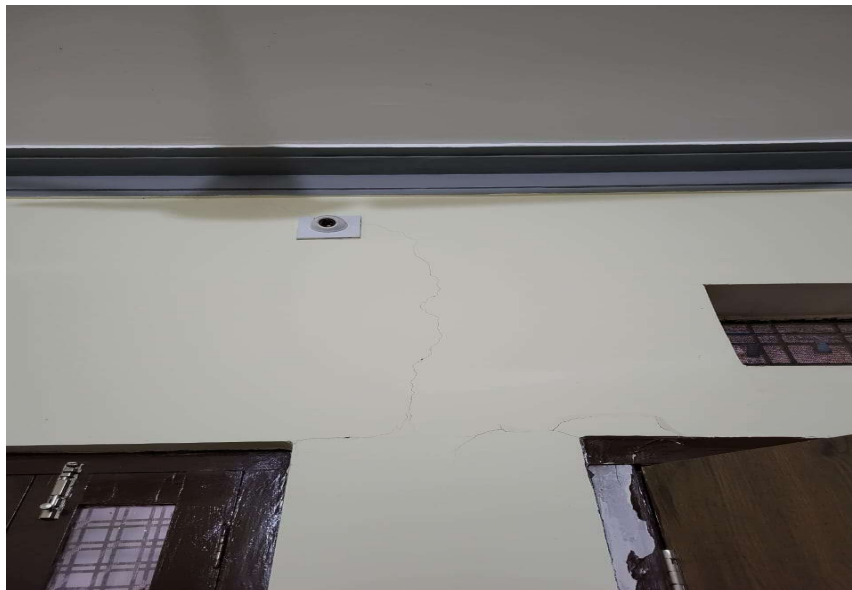
Image 8: Cracks on walls due to blasting in the mines
