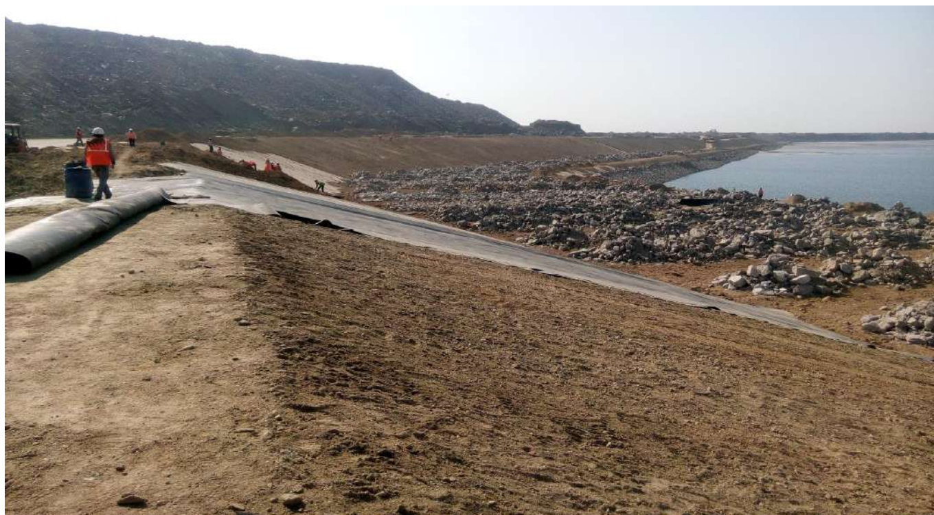
HDPE laying in tailing dam
