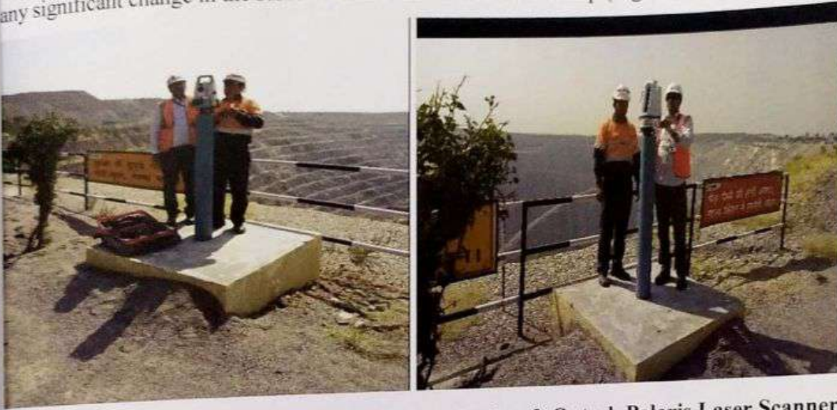
Fig. 11 - Monitoring observations with Total Station & Optech Polaris Laser Scanner
