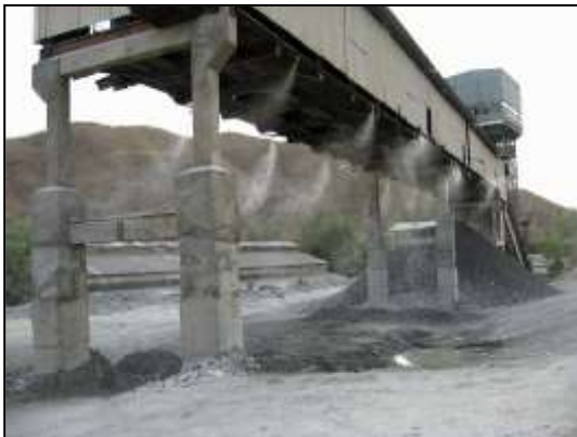
Mochia Coarse Ore Stockpile
