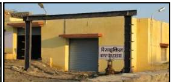
Recycling Water Pump House
