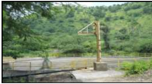
2,000 m3 Capacity Water Reservoir
