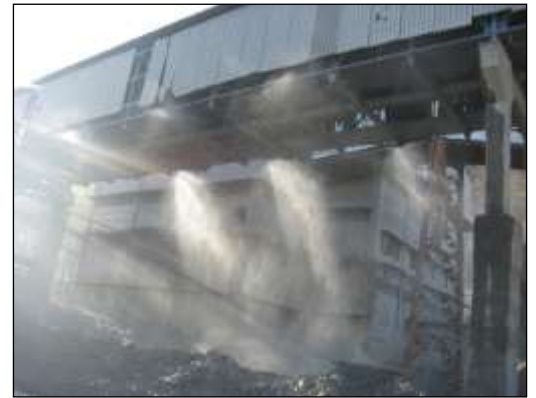
Balaria Coarse Ore Stockpile
