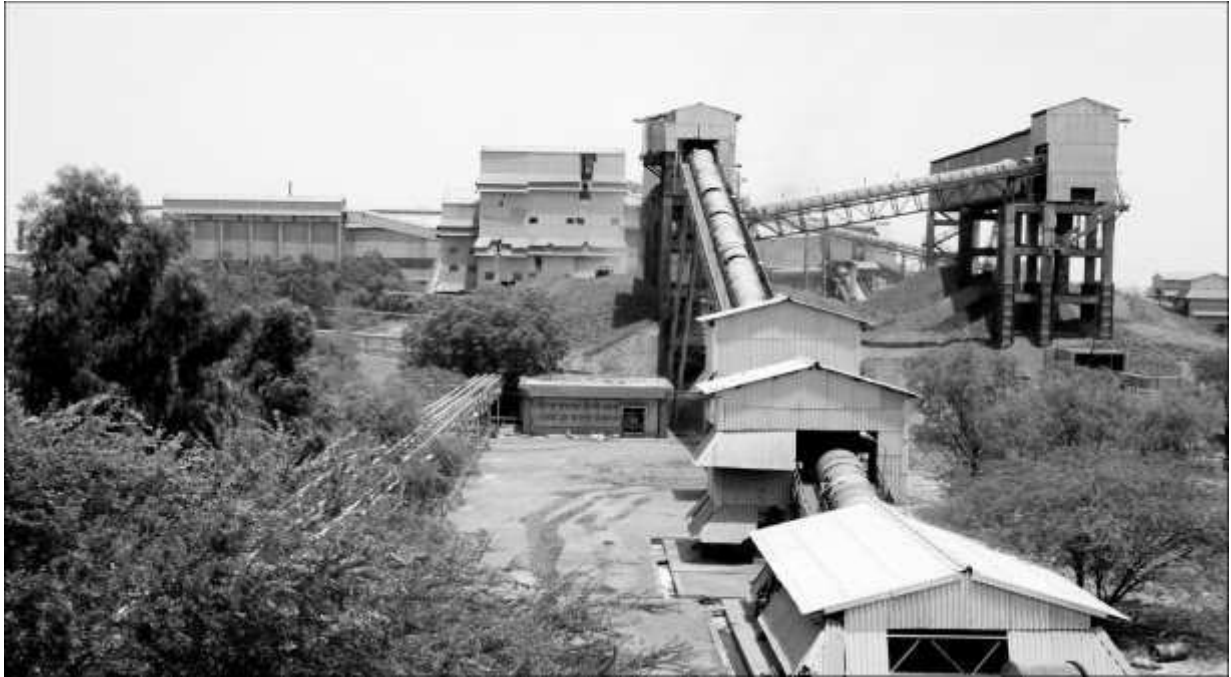
Covered conveyer belt
