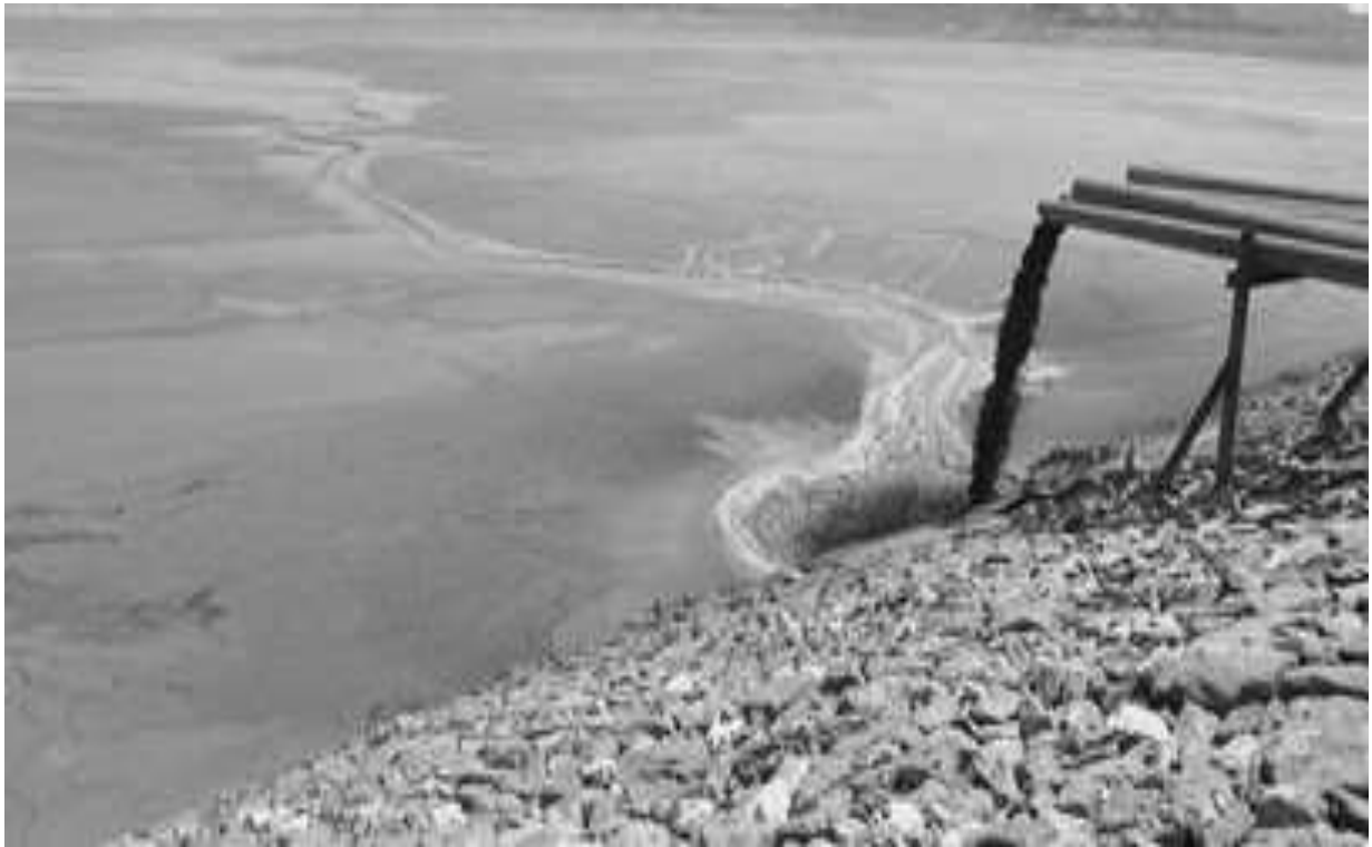
Tailing close pipe line
