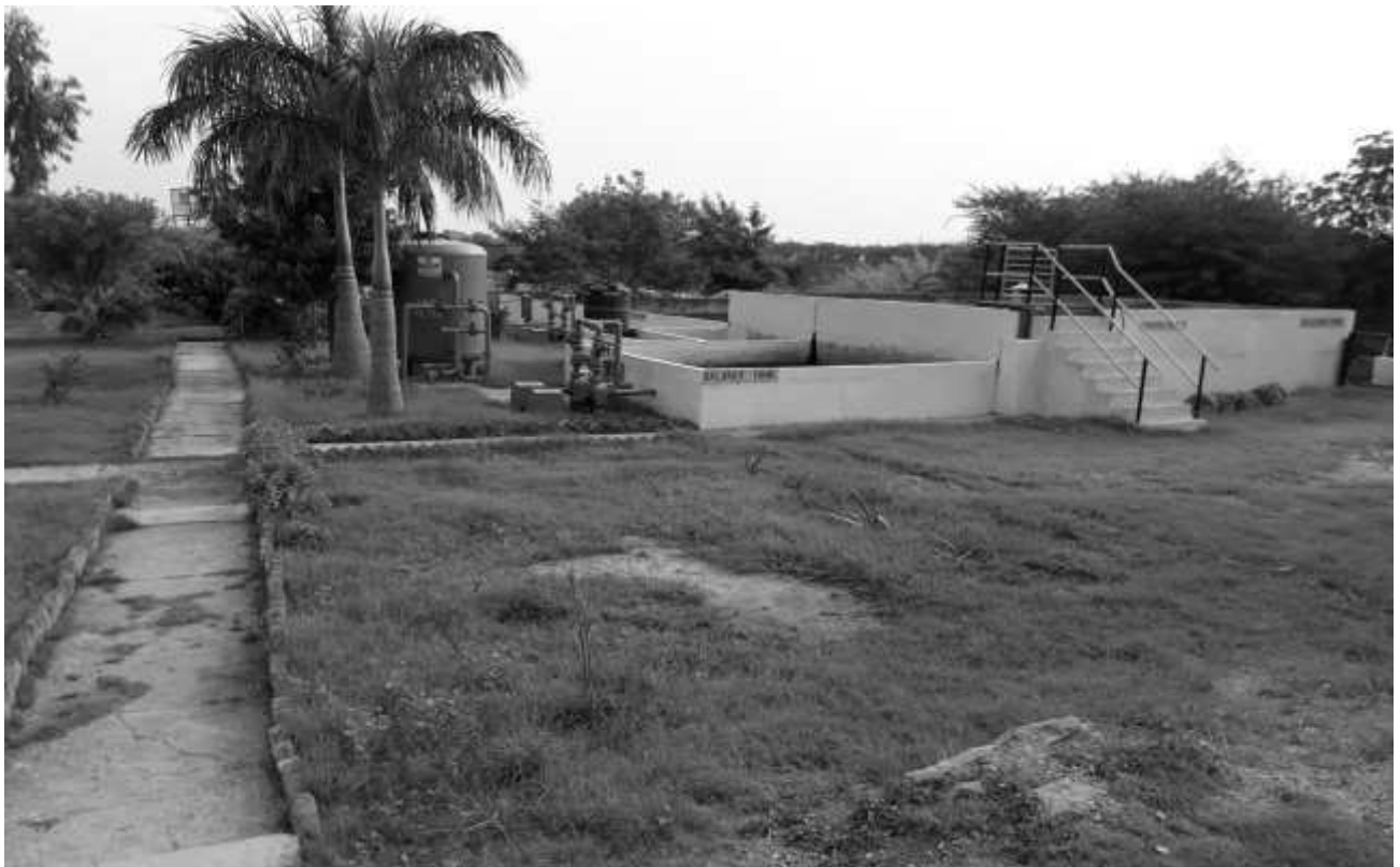
STP (300KLD) in plant premises
