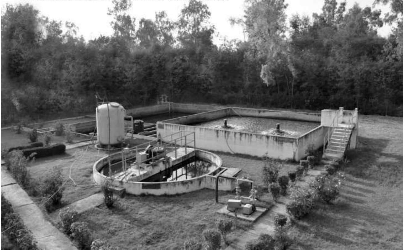
STP (425KLD) in plant premises
