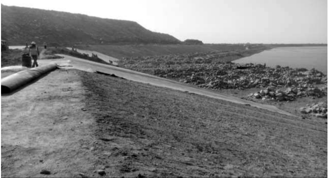
HDPE laying in tailing dam
