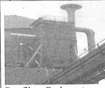
Bag filter, Cyclone at Coal Crusher
