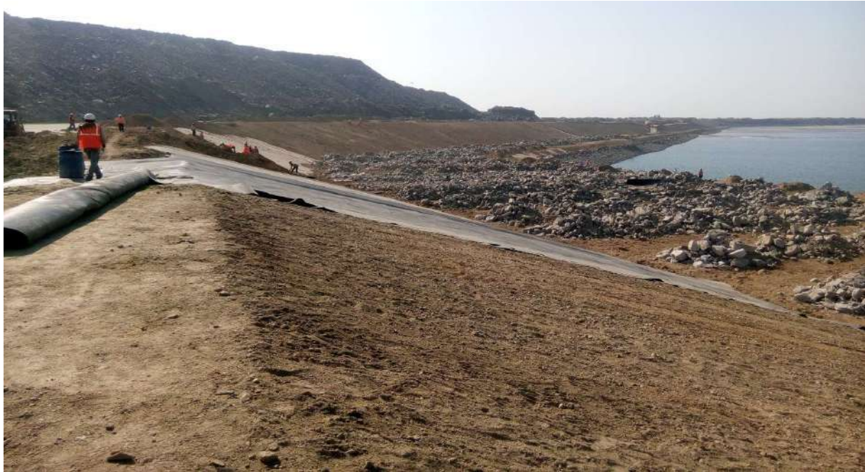
HDPE laying in tailing dam
