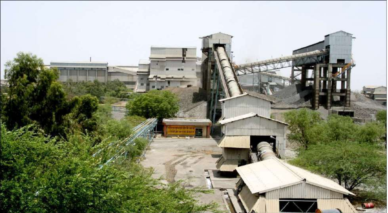
Covered conveyer belt
