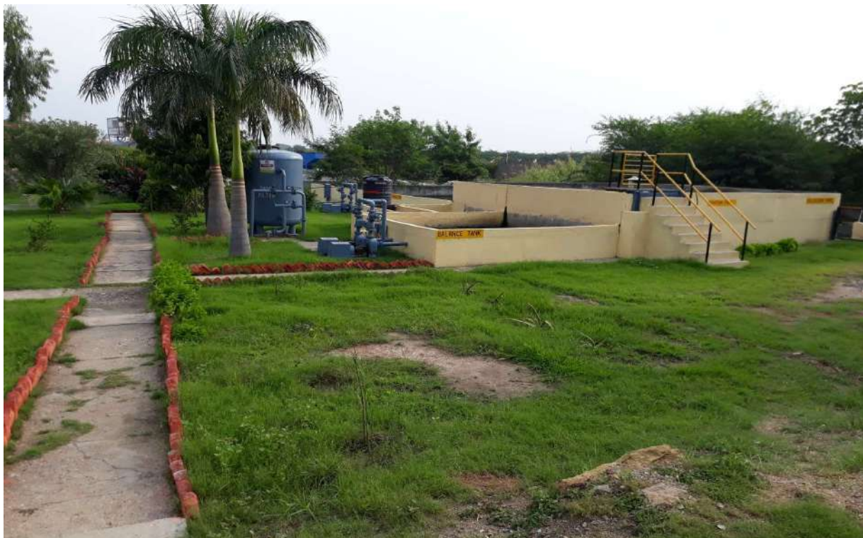
STP (300KLD) in plant premises
