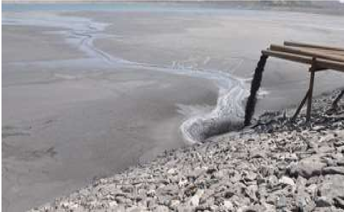
Tailing close pipe line
