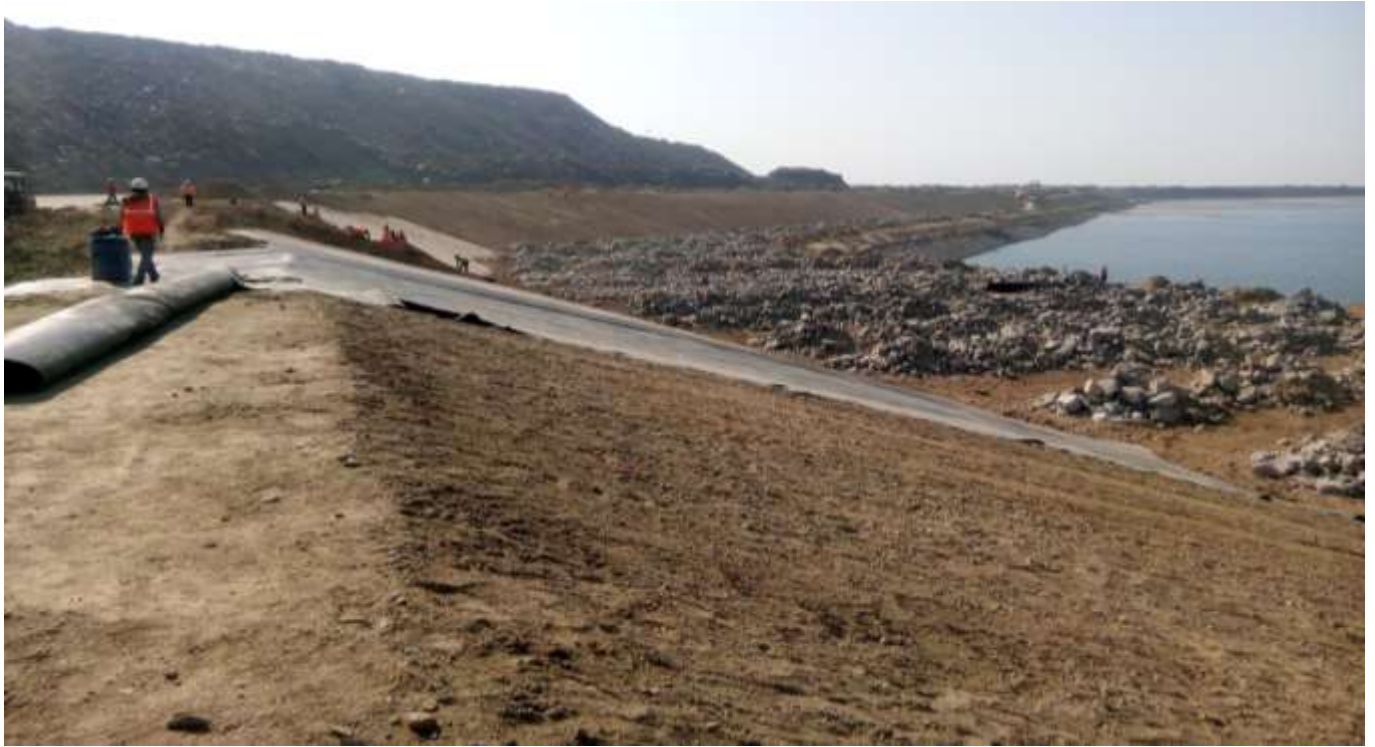
HDPE laying in tailing dam
