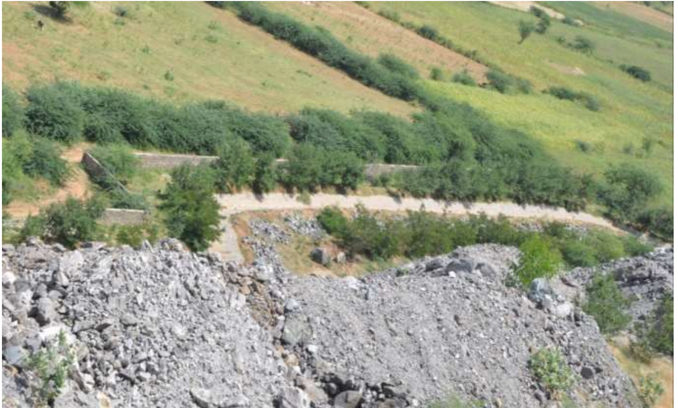
Garland Drain Photo
