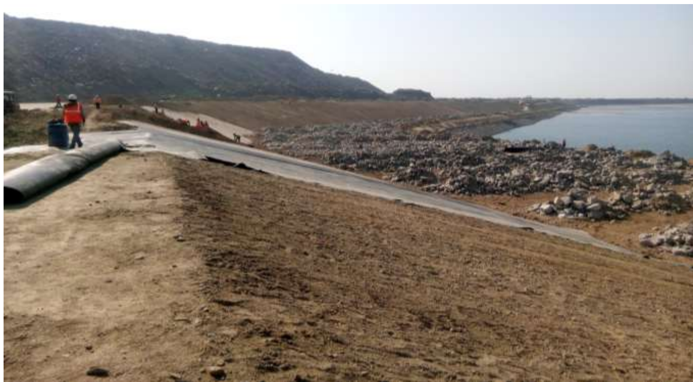
HDPE laying in tailing dam
