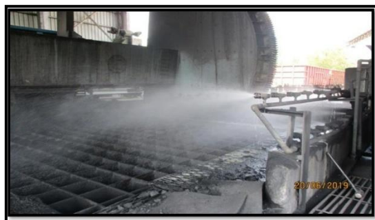
Sprinkler at coal transfer point
