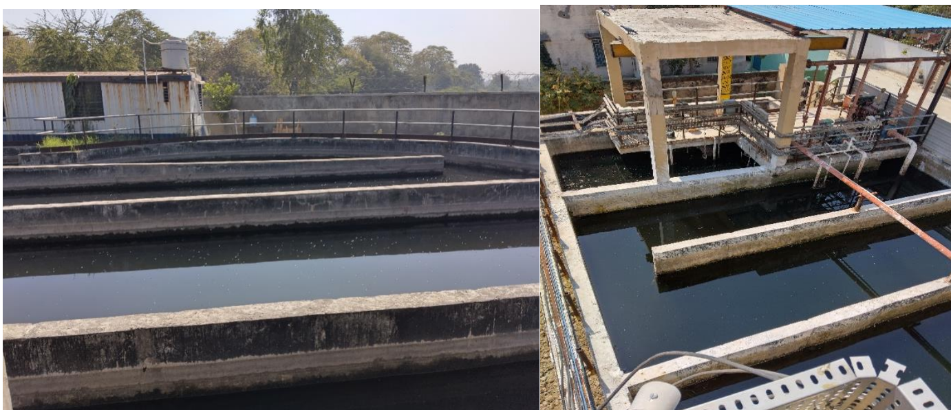
Figure 11 - Chlorination happening in CCT Tank
