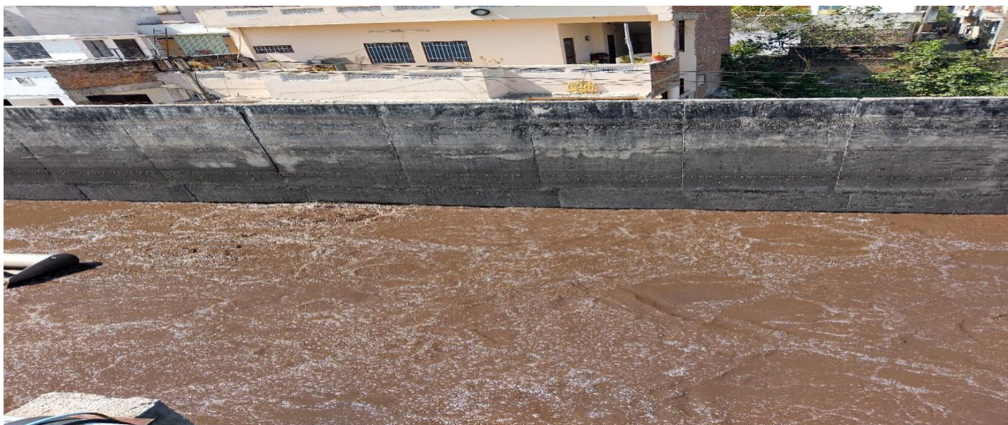
Figure 8 - Aeration happening through diffusers
