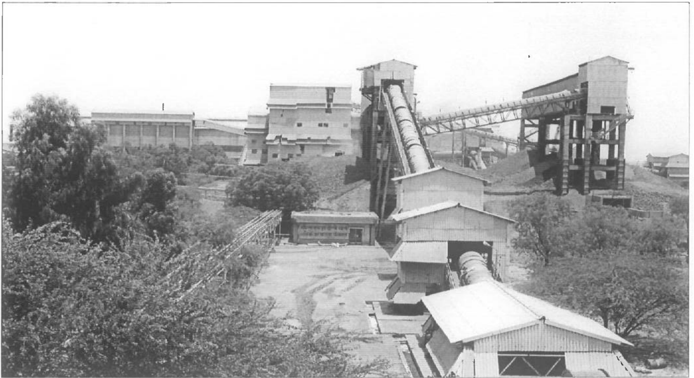
Covered conveyer belt
