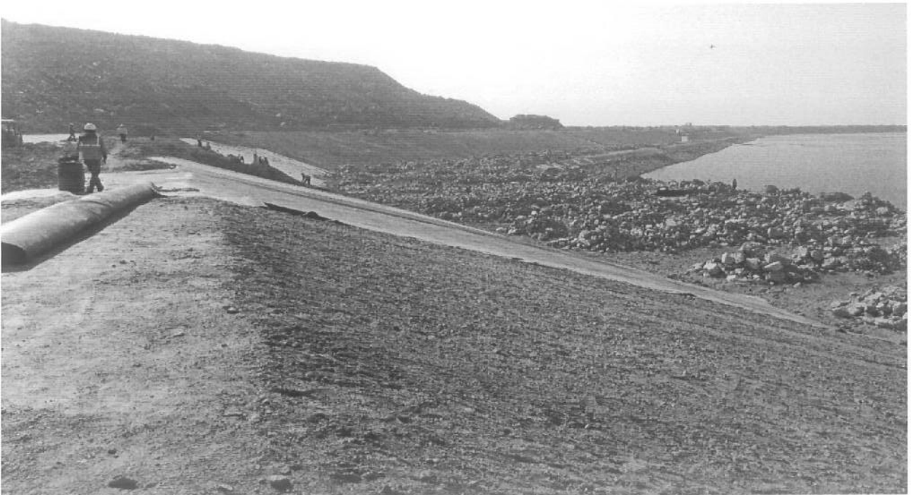
HDPE laying in tailing dam
