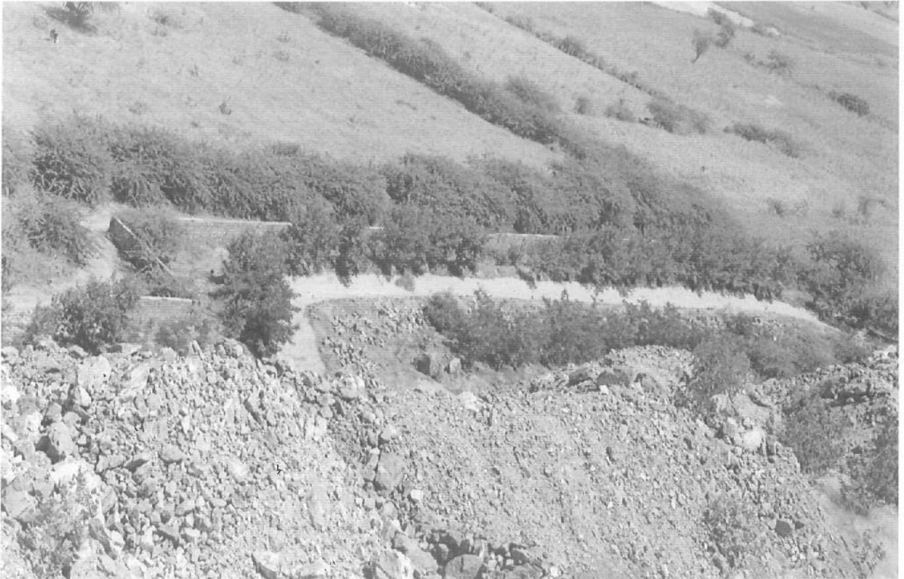
Garland Drain Photo
