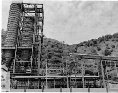
Hydro Fill Plant
