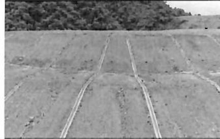
Tailing Embankment Drain
