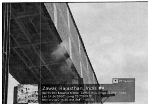
Water Mist Sprinkler at crusher
