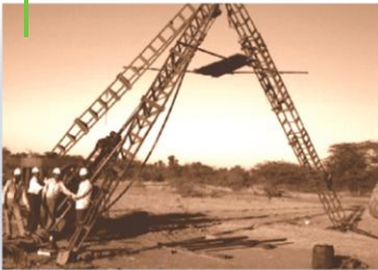
Conventional drill rig
