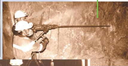
Drilling by hand-held hammer
