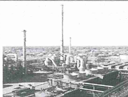
DCDA Gas Conditioning Plant (GCP) with 100 mt Stack Height
