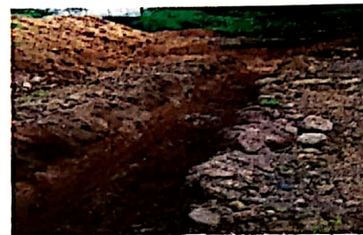
GARLAND DRAINS AROUND WASTE DUMP
