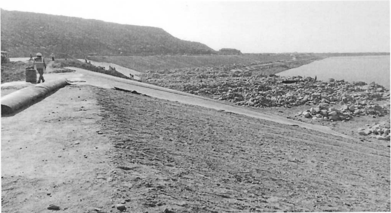
HDPE laying in tailing dam
