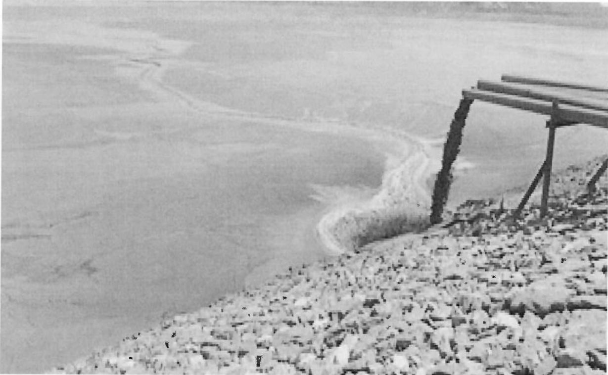
Tailing close pipeline
