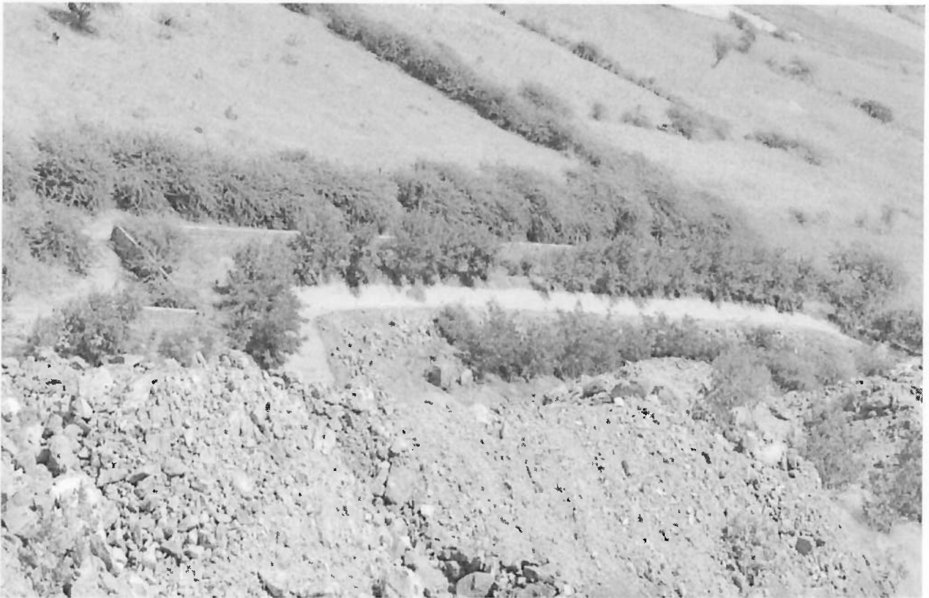
Garland Drain and Retaining Wall Photo
