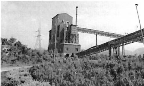
Covered conveyor belt
