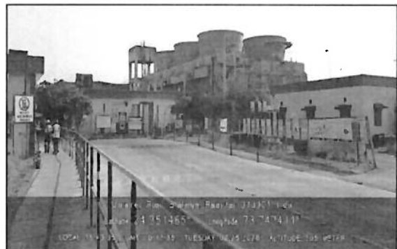
Concrete roads in Plant
