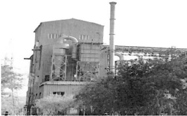
Coal Crusher Building
