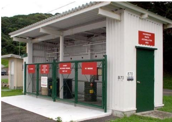
A typical secure, sheltered, storage area waste types
