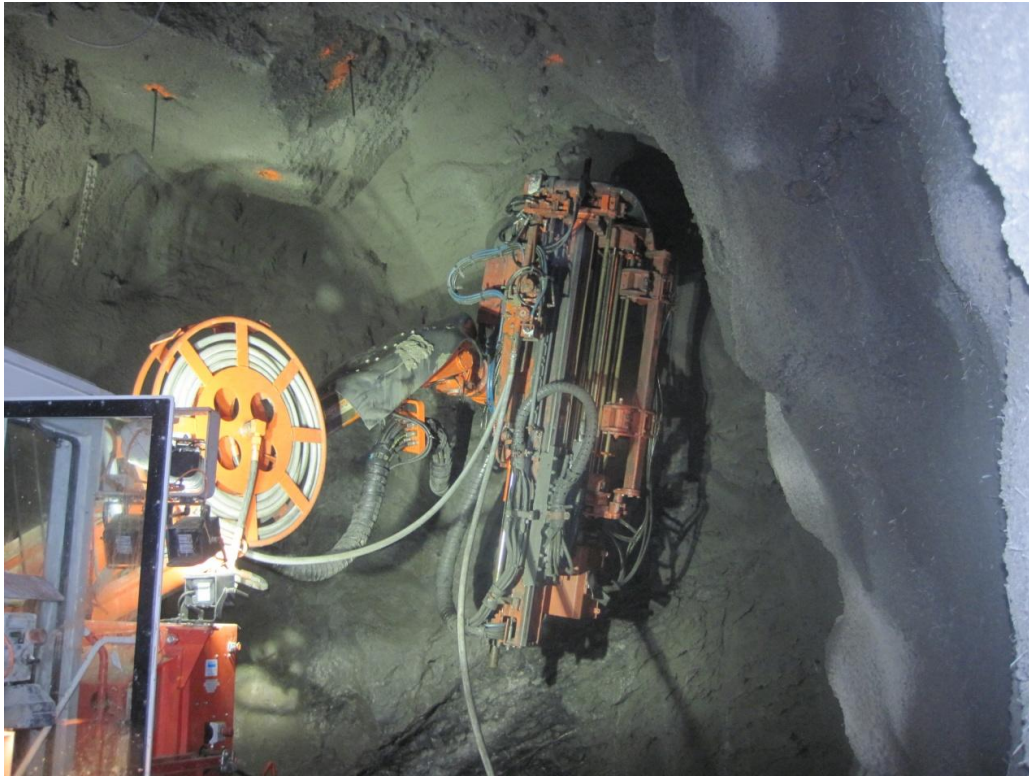
Figure 12: Installing cables with the Tamrock DSC-420
