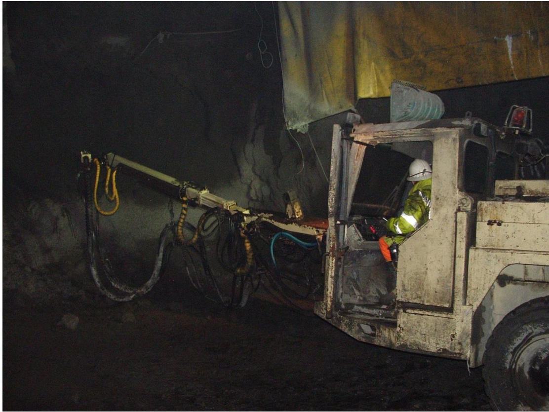
Figure 11: Shotcrete application with Spraymec
