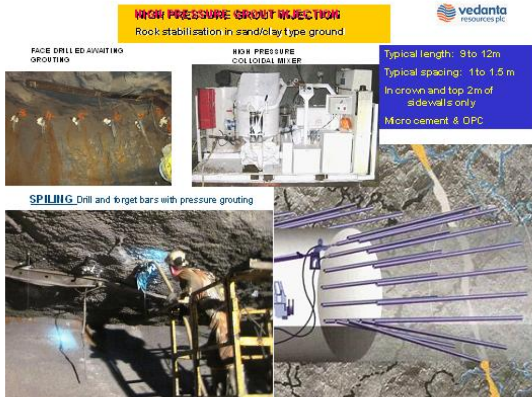
Figure 14: High pressure grout injection
