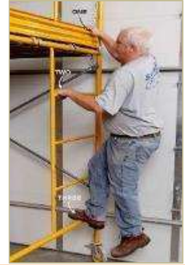
Figure 54: Using the end frames of an H-frame scaffold for climbing
