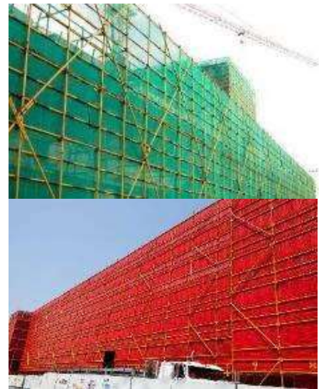
Figure 36: Examples of cloth type and metallic mesh type Perimeter Containment Screens
