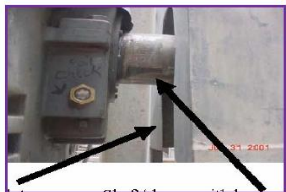
Slot opening is too large. Shaft/sheave with key way is not sufficiently guarded.
