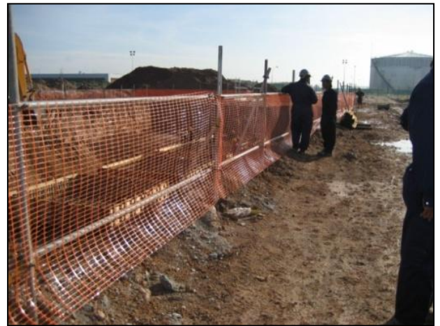
Barricading around Excavation
