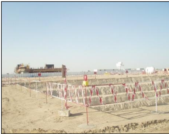
Barricading around Excavation
